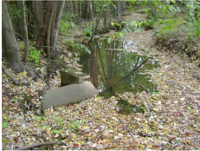
Photograph 5.1: Woodland Elementary School Outfall with broken headwall and exposed discharge pipe, October 22, 2008.
