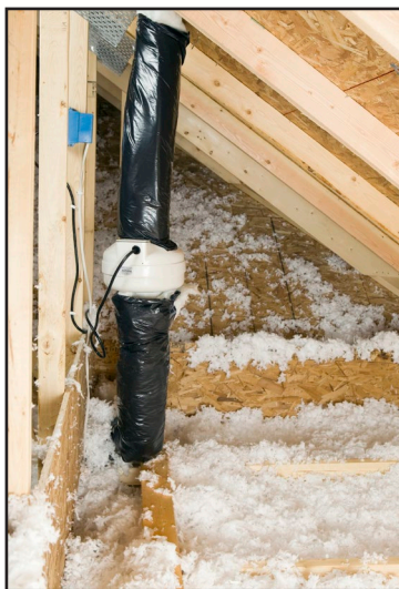
An active radon ventilation fan with black pipe insulation. The fan runs continuously, depressurizing the area below a concrete slab in the basement floor. Radon gas is captured by a drain tile below the floor and extracted from the house via the fan shown here. Credit: istockphoto.com/BanksPhotos
