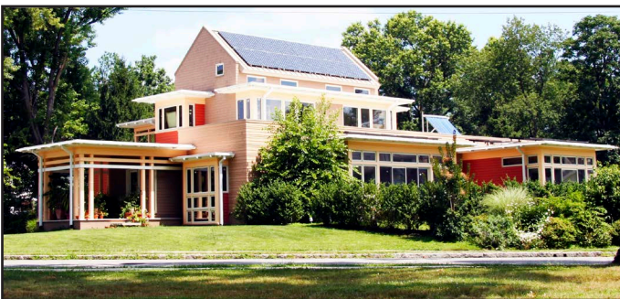
Half Moon House in downtown Madison, NJ, was one of seven area homes included in GSWA's first-ever home and garden tour in May 2014. This particular home boasts a number of green features, including a geothermal well, a solar panel array, low-VOC interior finishes, and cedar shingles certified by the Forest Stewardship Council. Credit: Courtesy of C. Kellogg
