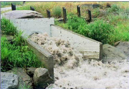
One of the main conduits of non-point source pollution: a stormwater outfall shown above delivers water and pollutants from a wide area, such as residential communities and parking lots.
