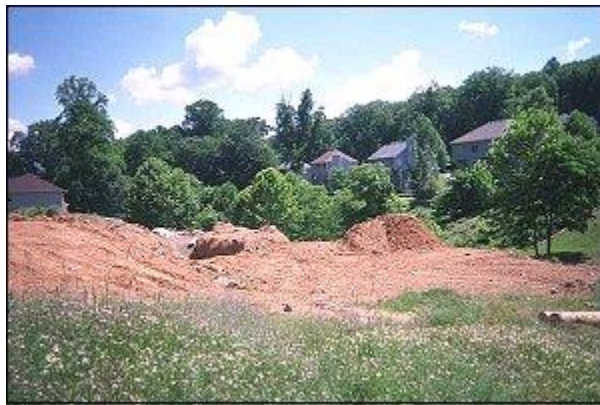
The potential for excess sediment to enter streams is greatest during site preparation and construction of a new development.
