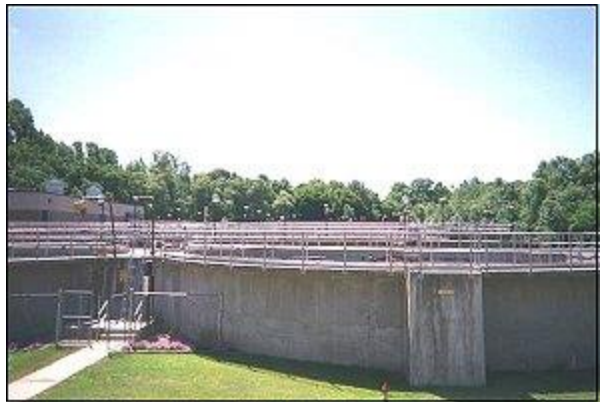
Settling tanks at the Woodland Sewage Treatment Plant in Morris Twp.
