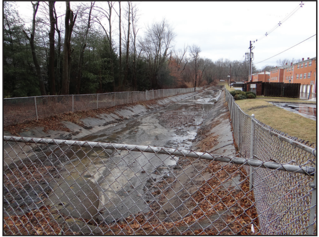
Figure 3: Chatham Hill detention basin clean with vegetation all cut back
