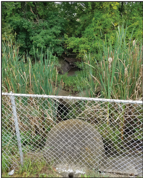
Figure 2: Chatham Hill detention basin with standing water blocked by vegetation.
