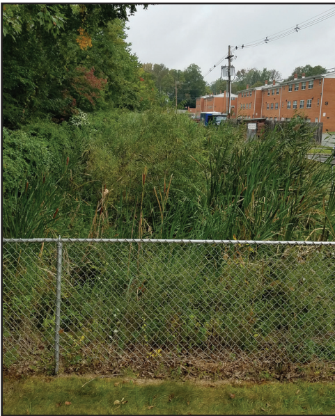
Figure 1: Chatham Hill detention basin filled with cattails and other vegetation.
