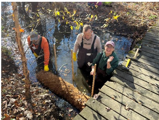
Sandra with volunteers installing a coir log to protect the bank of the Silver Brook
